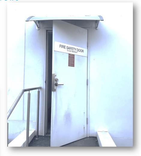
Passive Fire Protection = Barrier or Shield to stop spread of fire
